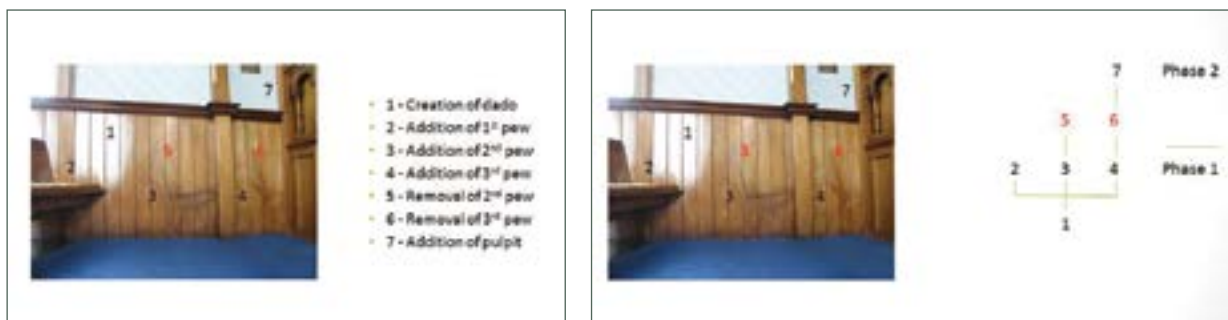
Figs. 8 and 9. A written summary of stratigraphic units or 'events' (above) and a phased, stratigraphic diagram illustrating the chronological relationships between these events (below) (Martin Jones IMG008 and IMG009).
