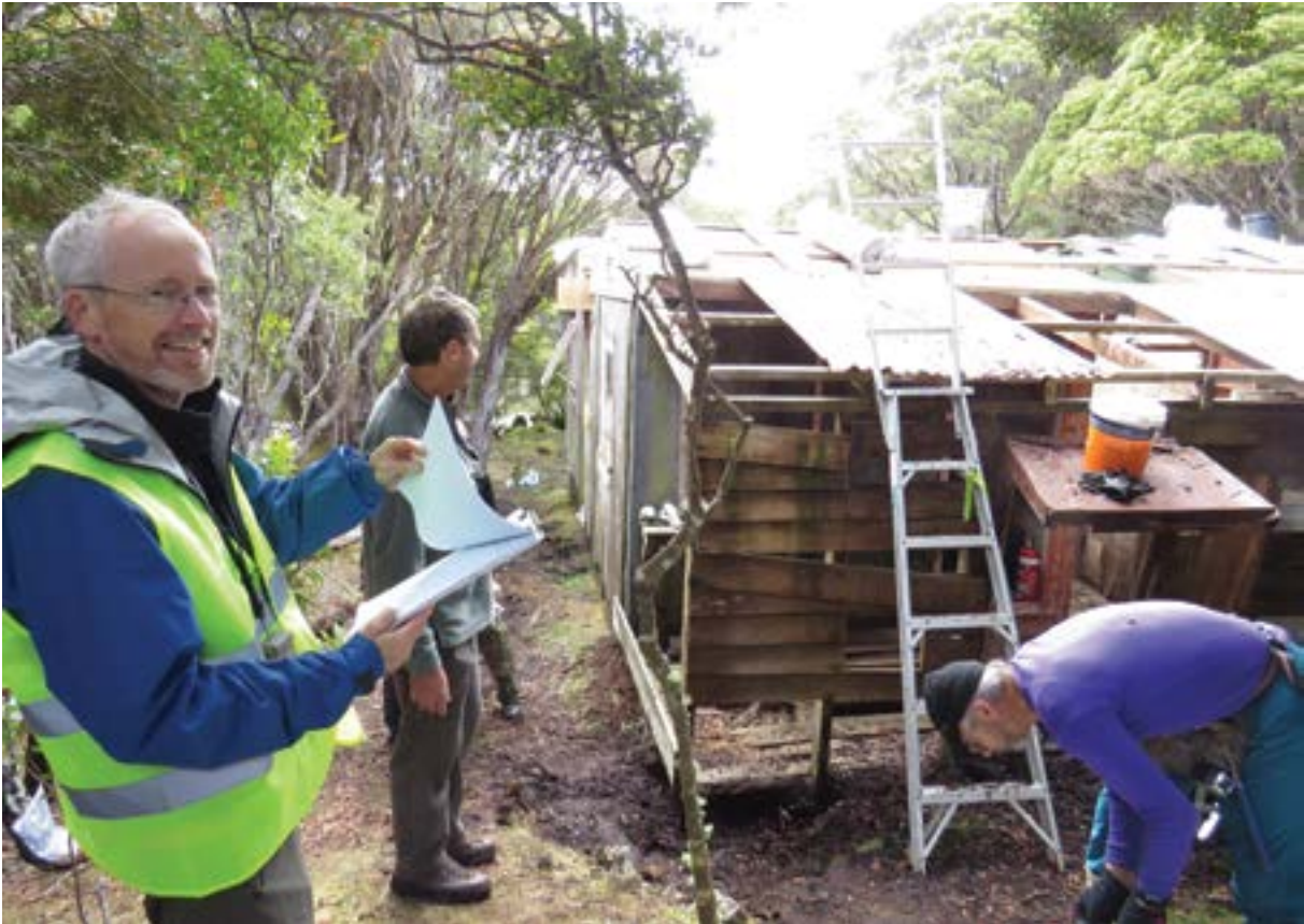
Fig. 6. Coastwatcher Hut works on Auckland Islands (HNZPT IMG005)
